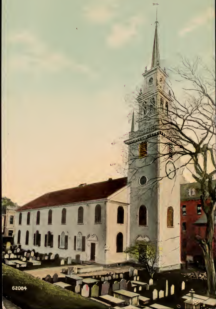
Exterior of Trinity Church, Newport, R.I.
